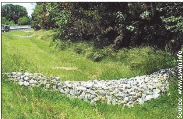
Vegetated swale on roadside with check dams installed.
